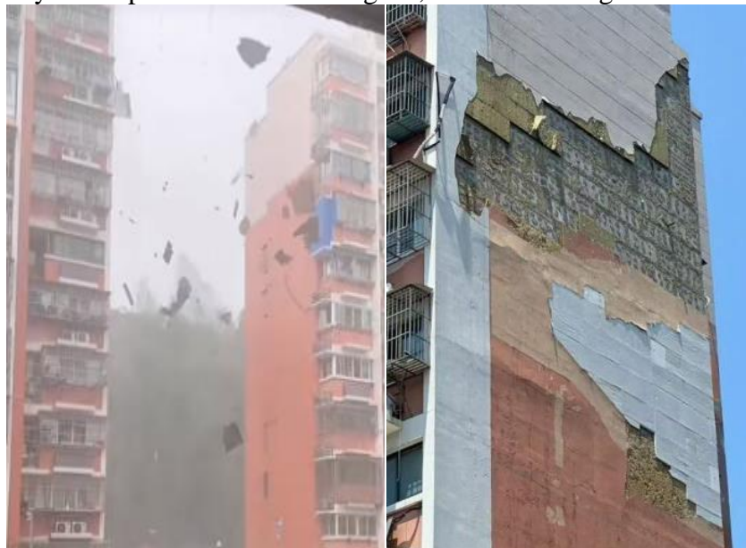
Figure 2 External Wall Detachment of the Rock Wool Thin-Plaster System
