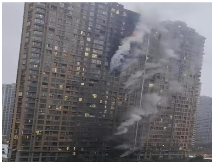
Figure 1 Fire spread in the Polyurethane Thin-Plaster External Wall System
