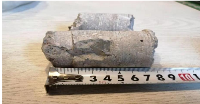
Figure 6: Crack depth measurement of the second set of drill core sampling
