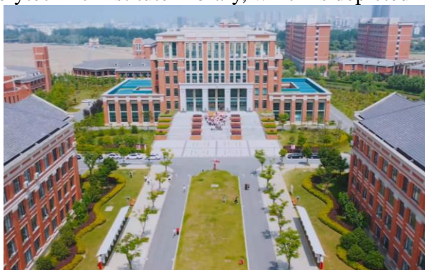
Figure 1: Jiaxing Nanyang Polytechnic Institute Library
