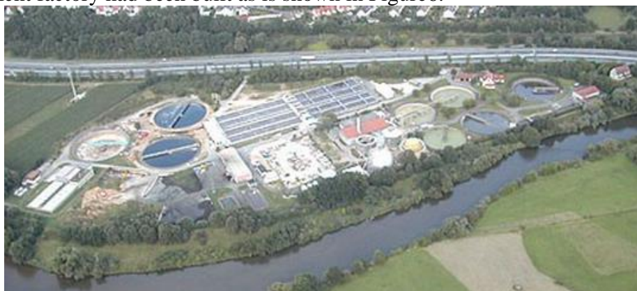
Figure 6: The sewage treatment factory of Erlangen
