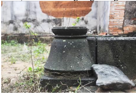
b) Foundation pillars in Suer village
