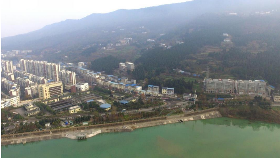
Figure 1: Overall View of Landslides after Small Earthquakes
