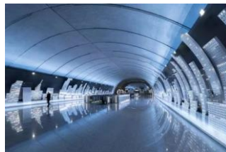
Figure 1 The Wuzhong Rd. Metro Station in Shanghai
