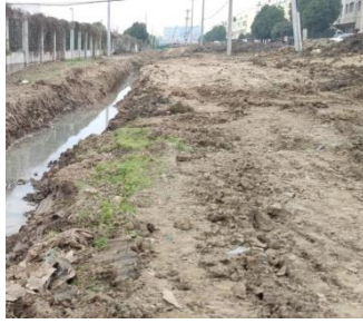
Figure 4: Drainage and air drying of the subgrade
