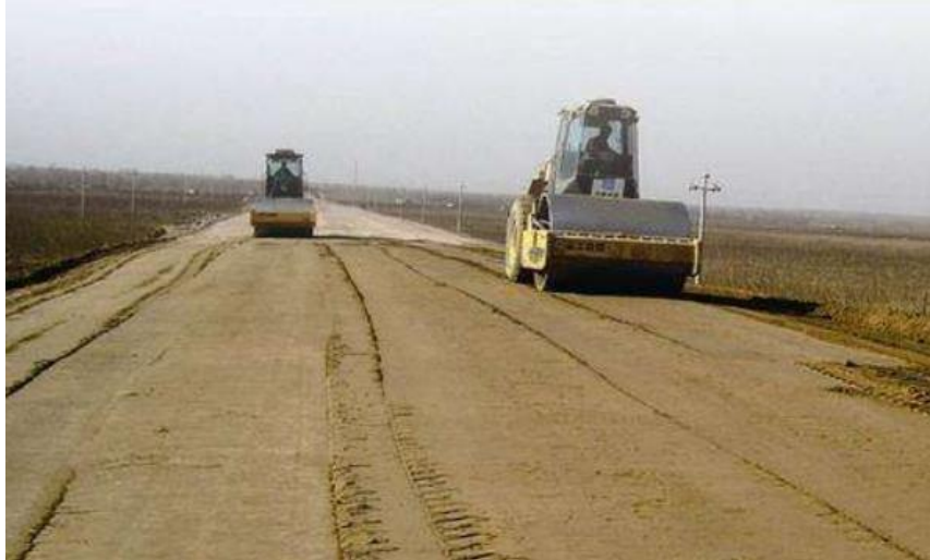
Figure 2: Pavement compaction.
