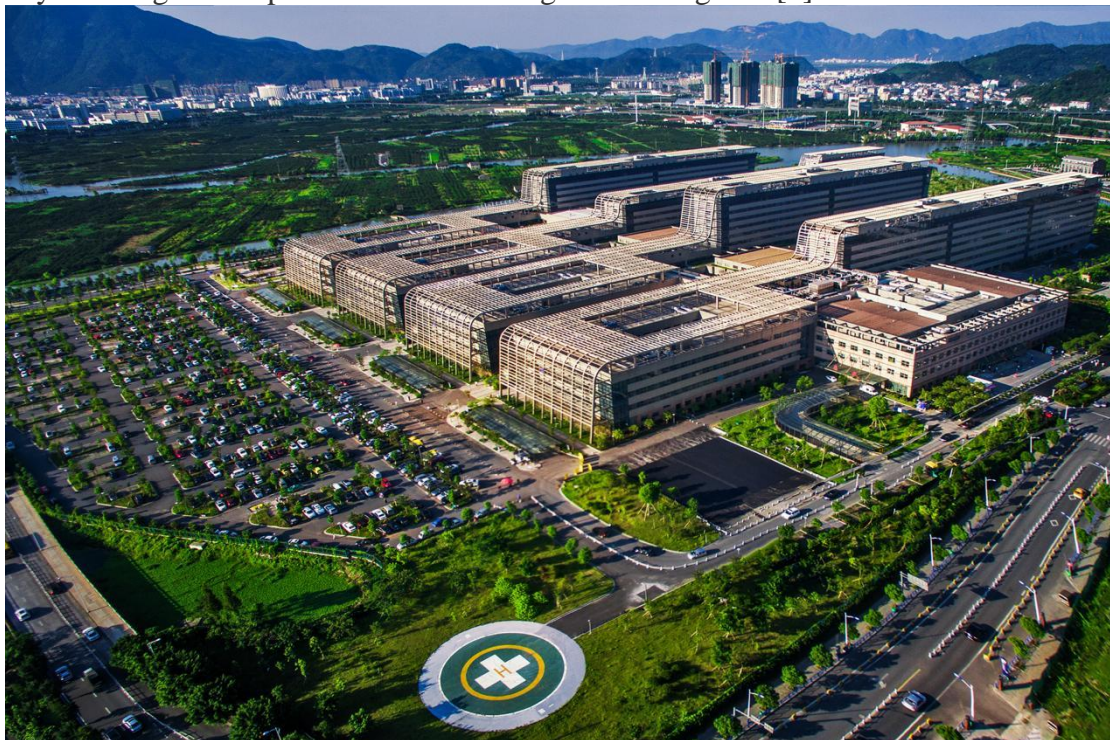
Figure 1 Overview of the new hospital
