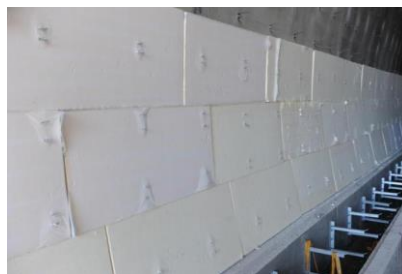
Figure 1: Insulation board laying
