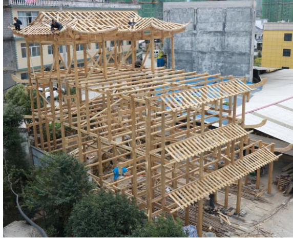
Figure 1: The wooden frame of Tujia Stilted Building
