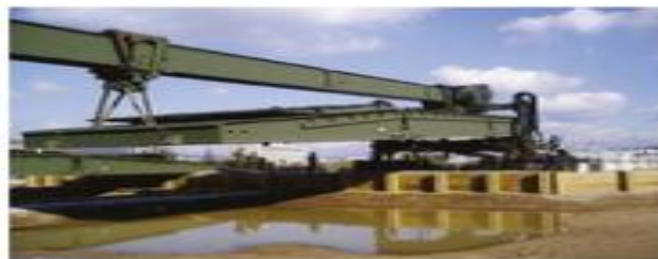
Figure 3: Dry Support Bridge (DSB)
