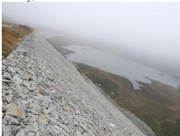
Figure 6: Photo of embankment slope of Linfeng Avenue, Yilong New District
