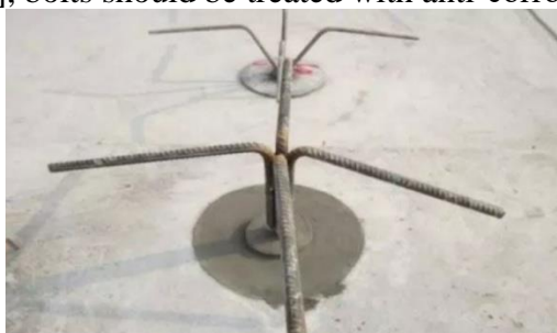
Figure 1: Schematic diagram of main reinforcement of anti floating anchor rod
