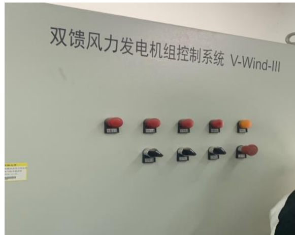
Figure 5 Control system of double-fed wind turbines
