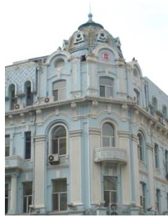
Figure 8: Building with masonry
