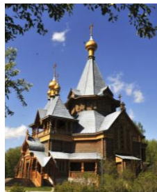
Figure 6: Central Street Russian Architecture
