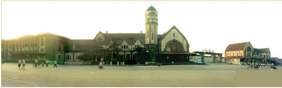
Figure 1: Jinan Old Railway Station
