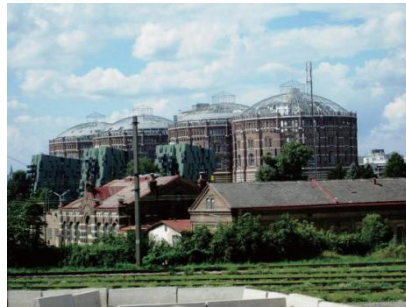
Figure 5: Reconstruction of Gas Storage Tank with Brick Outer Wall in Vienna
