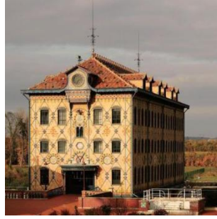
Figure 4: Renovation of the McNair Chocolate Factory
