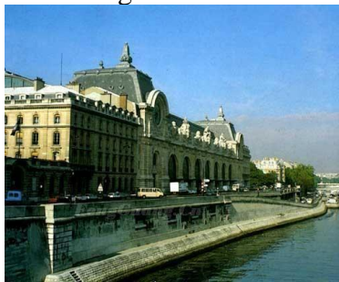
Figure 2: Orsay Train Station, France
