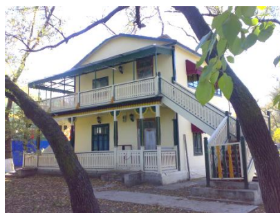
Figure 8: Corridor of a wooden building
