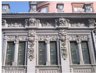
Figure 11: Columns between windows in Russian-style buildings
