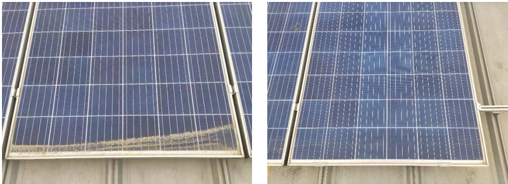
Figure 4: Comparison diagram of component dust accumulation
