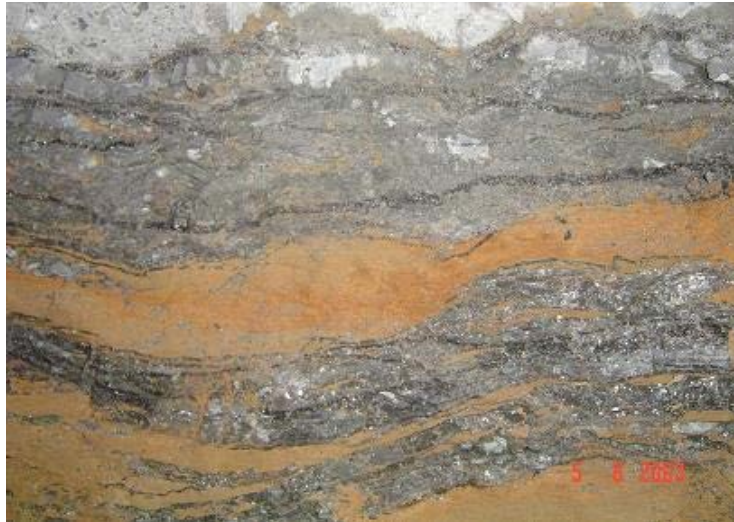
Figure. 7 Exposure groutingslurry in tunnel palm face
