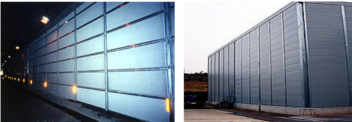
Fig. 1. Alporas aluminium foam sound absorption panels next to roads (left) or as buildings insulation (right) in Japan [6].
